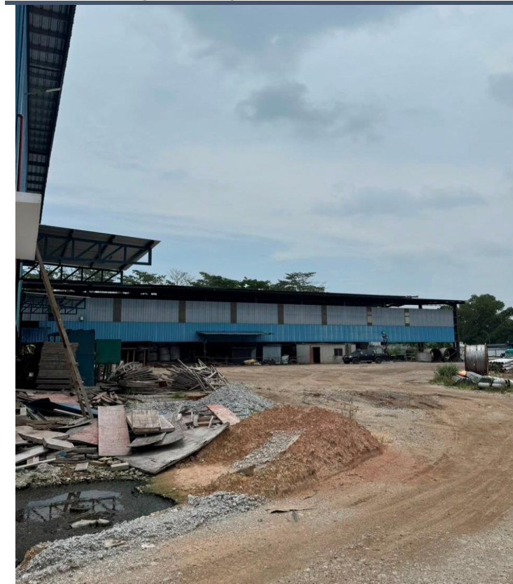
Figure #8 Existing building to be demolished for the new seven-storey CCV facility
