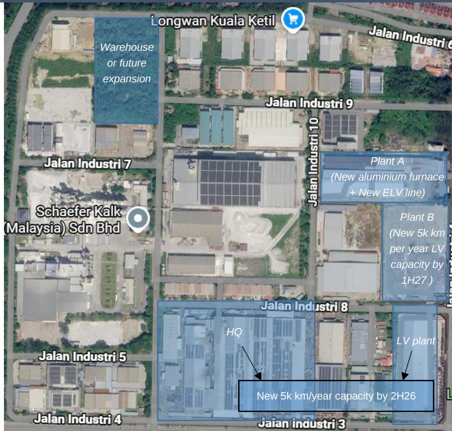
Figure #1 New 5k km/year located in HQ and its existing LV plant
