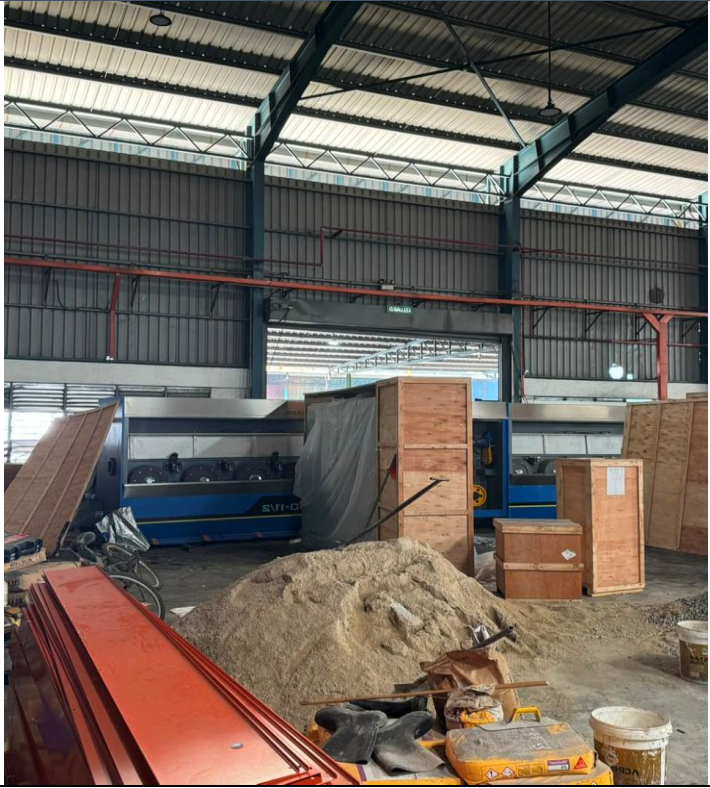
Figure #4 Ongoing on-site hook-up works for the new stranding line at HQ
